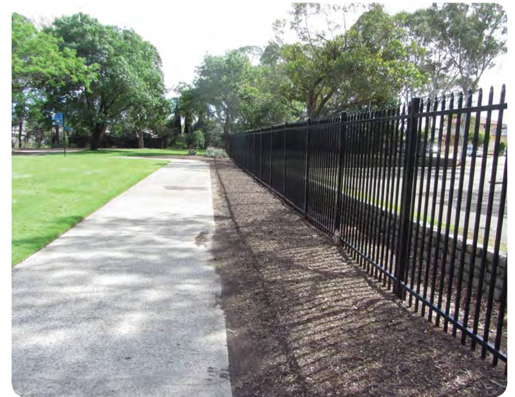
Chisholm Road boundary fence
