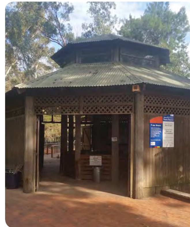
Entry structure to Fauna Park
